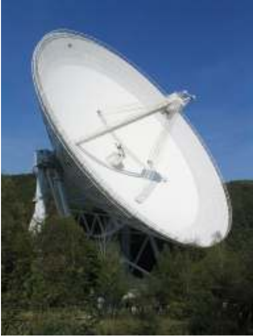
Fig. 2.2: The 100-m radio telescope at Effelsberg is operated by the Max-Planck-Institut für Radioastronomie (MPIfR) based in Bonn. It is one of the largest fully steerable radio telescopes in the world. The 21-cm receiver is installed in the primary focus cabin of the telescope.
